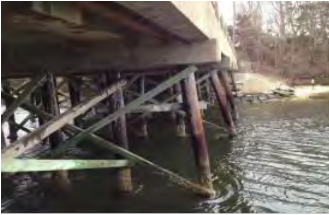
Bumps River Bridge
