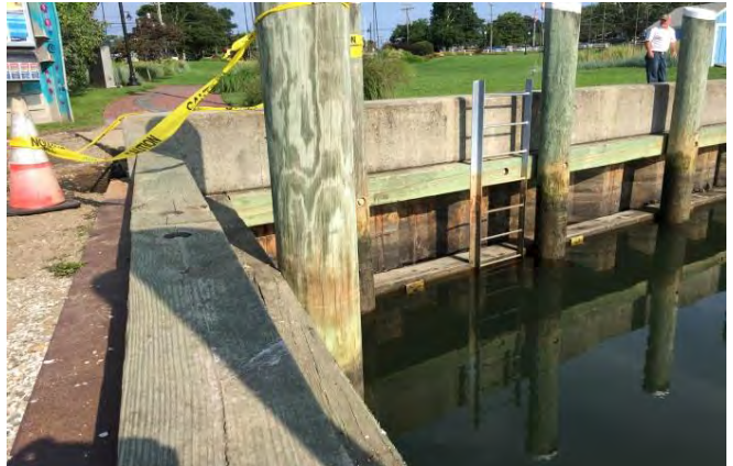
Gateway Marina Bulkhead
