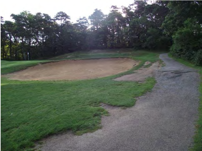
Hole #13 Deteriorating Cart Path & Bunker
