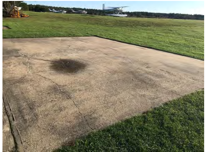
Cape Cod Air Field Underground Fuel Tank
