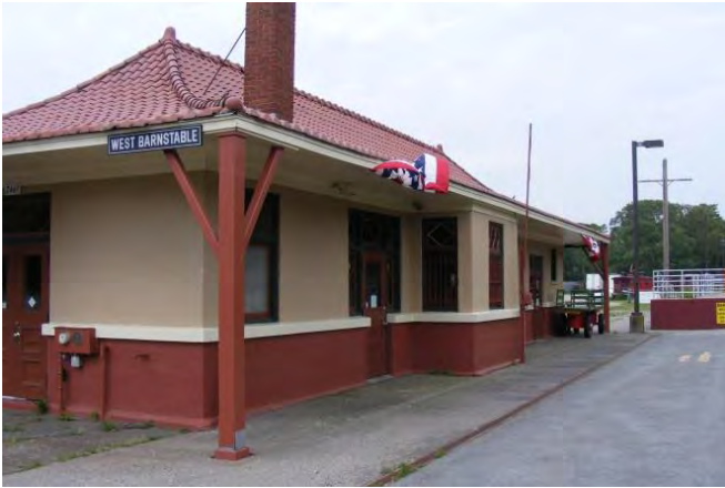
West Barnstable Railroad Depot
