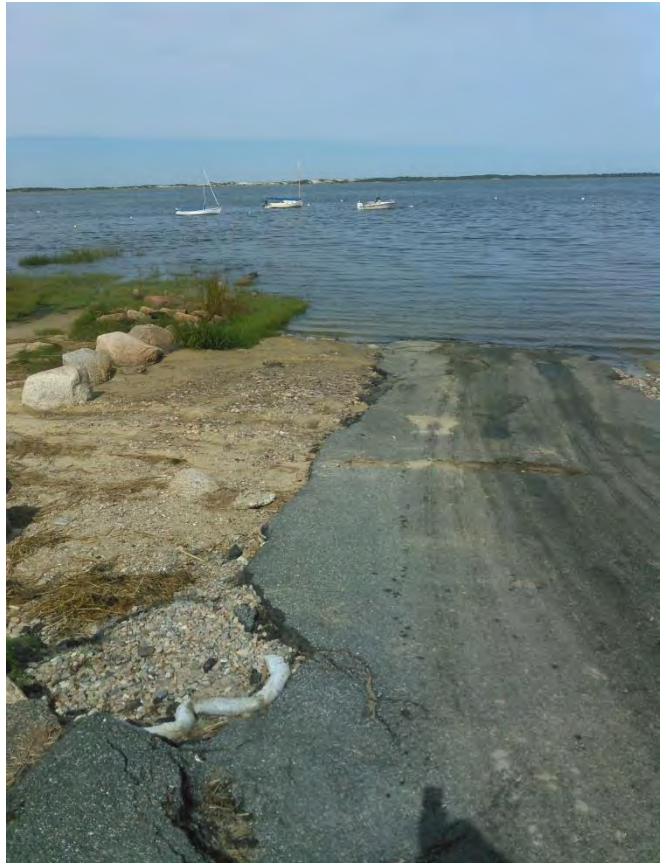
Scudder's Lane Boat Ramp
