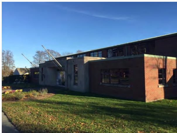
Armory Building Exterior
