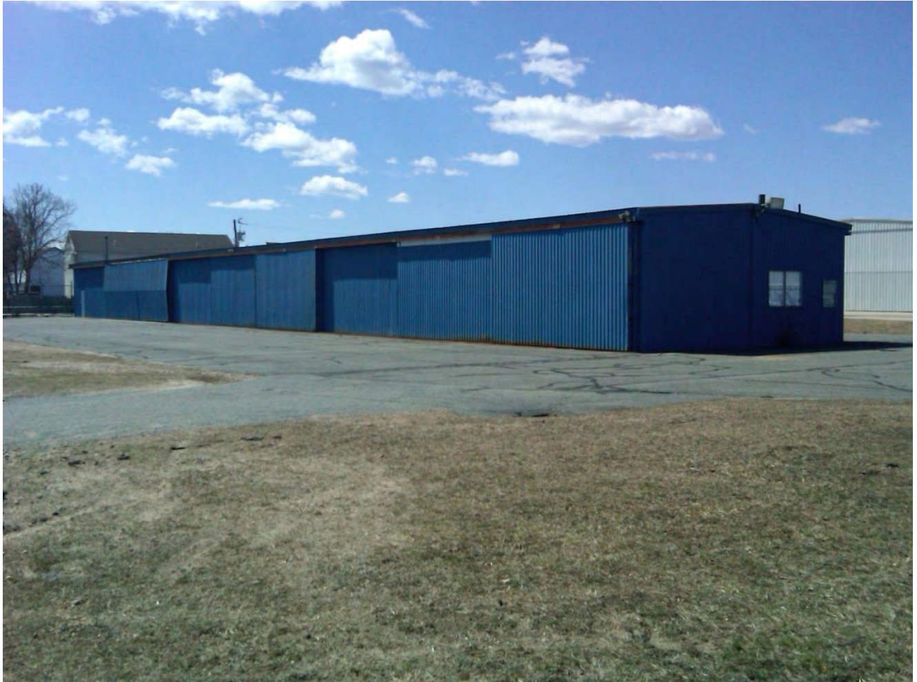
Airport-owned Existing T-hangar
