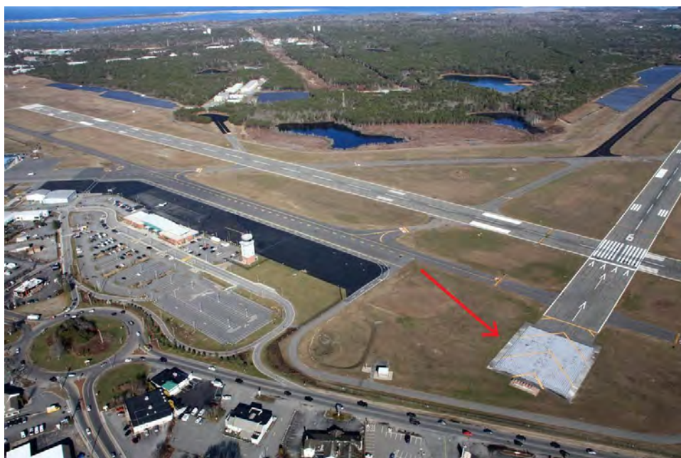
(Engineered Material Arresting System (EMAS) or Runway SAFE System)
