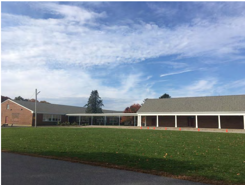
Hyannis West Elementary School Needs Roof Replacement
