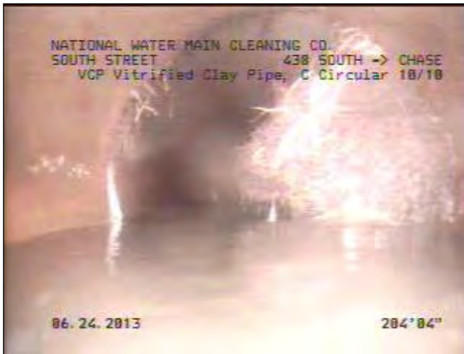
Sewer Pipe Root Intrusion
