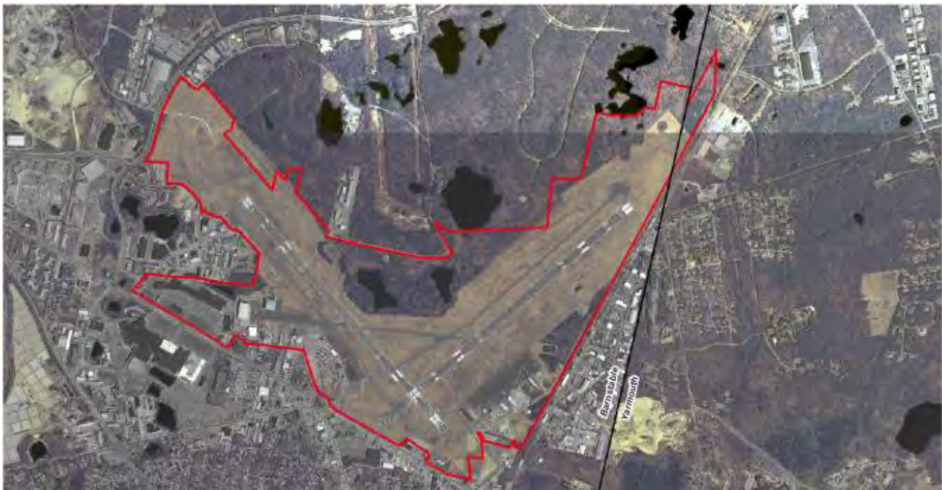
Airport Buffer Zone : Fencing and Vegetation
