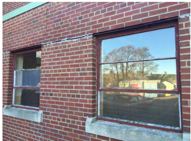
Armory Building Exterior
