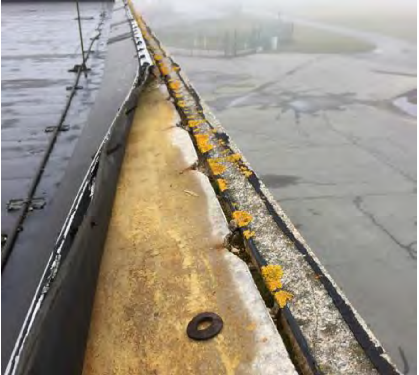
Roof of the Aircraft Rescue Fire Fighting (ARFF) Building
