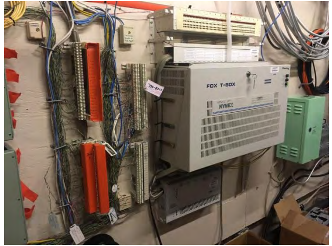
Existing High School Demark
