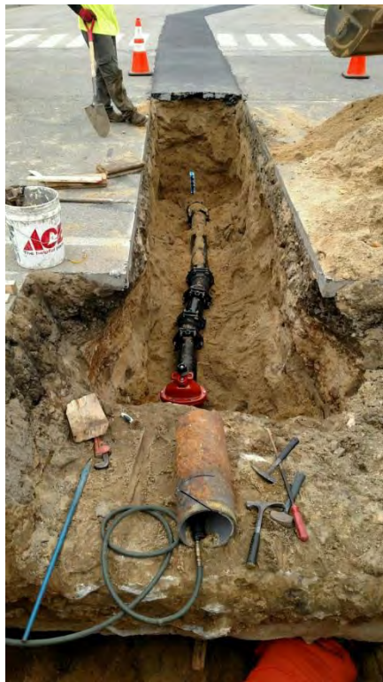
Water Pipe Replacement
