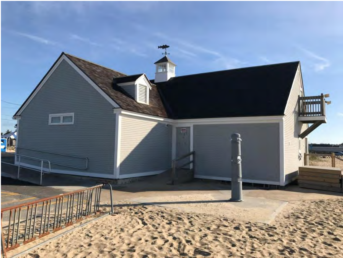
Craigville Bathhouse Septic Location
