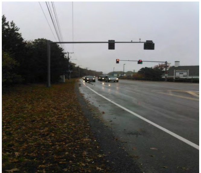
Location of Bike Path at Bearse's Way from Pitcher's Way to Route 28
